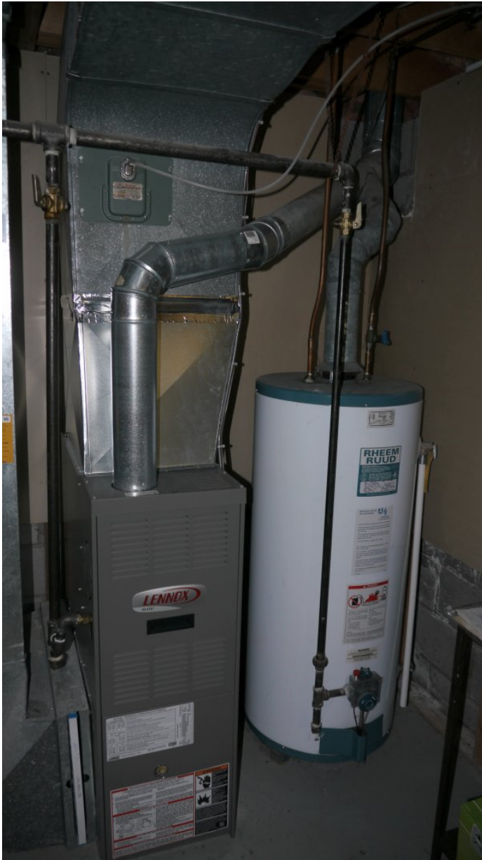
Furnace & Hot Water Tank
