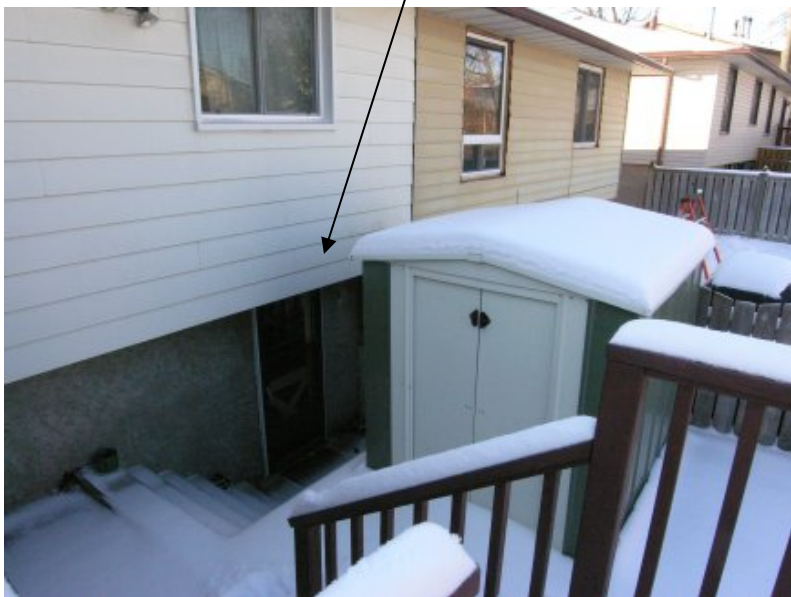
Lower Level Access Door
