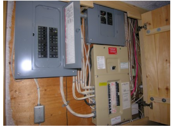
Electrical Distribution with Generator Panel
